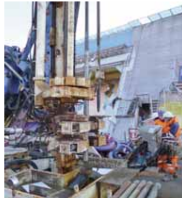
Carotaggi Core drilling
