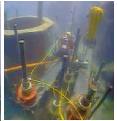
Tesatura e collaudo Testing and tensioning
