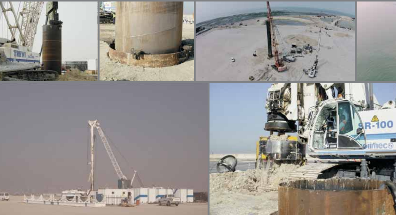
Area cantiere a terra / Onshore jobsite
